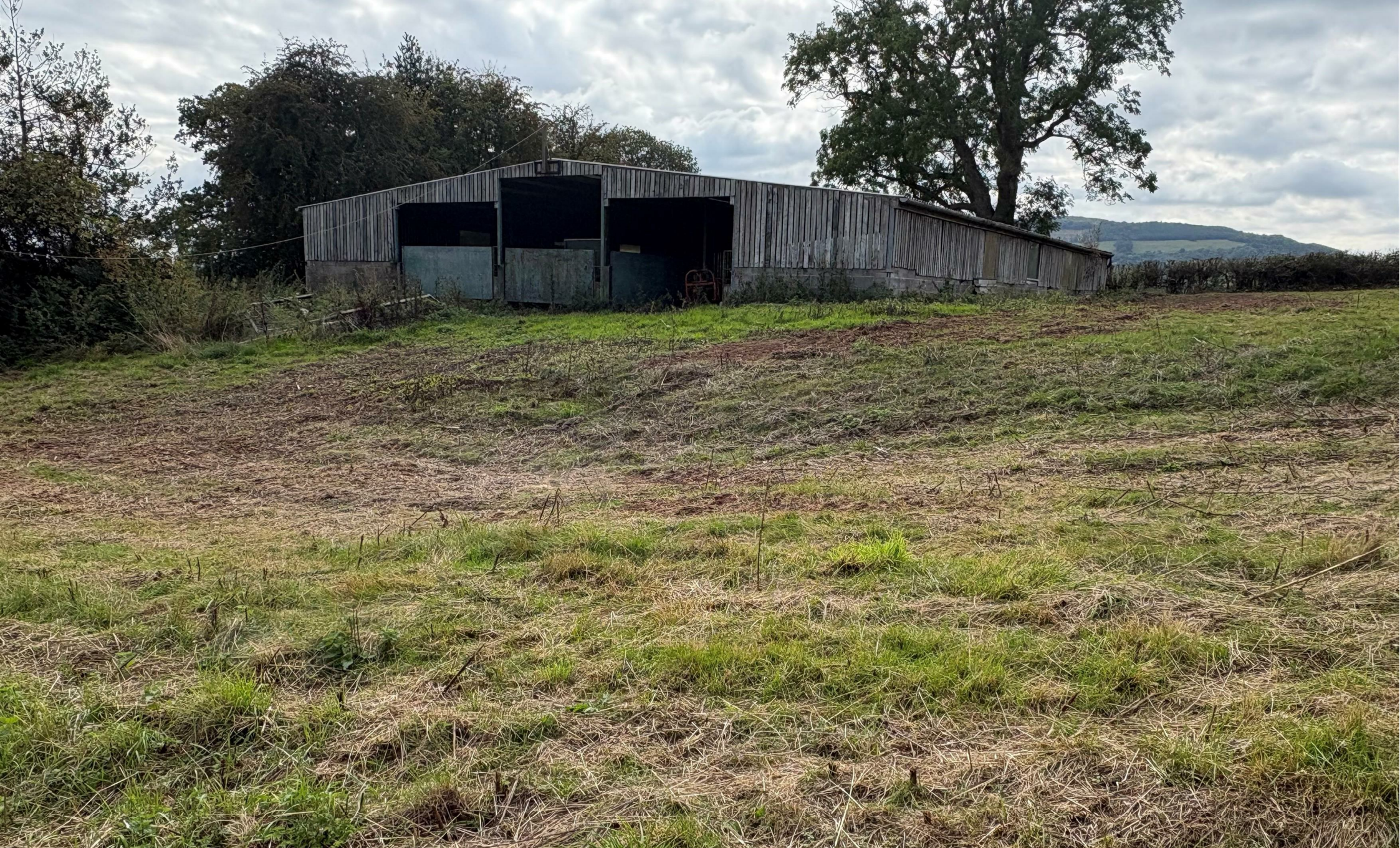
Barn for Conversion - 'Barn at Hyde Farm' Middleton Priors, Bridgnorth, Shropshire, WV16 6UR
